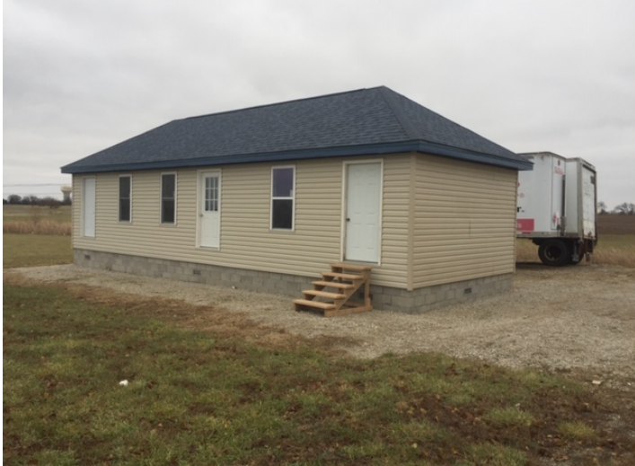
New energy training lab
