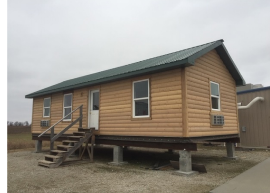
6 th cabin built by NCCC students
